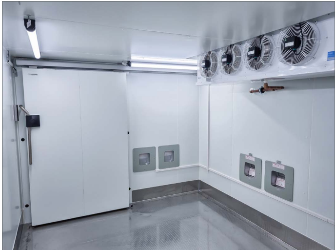
Lock with active -20 \text{ }^\circ\text{C} cooling
