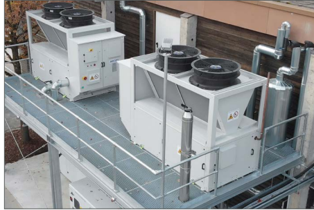
Water chiller with R290 from Secon
